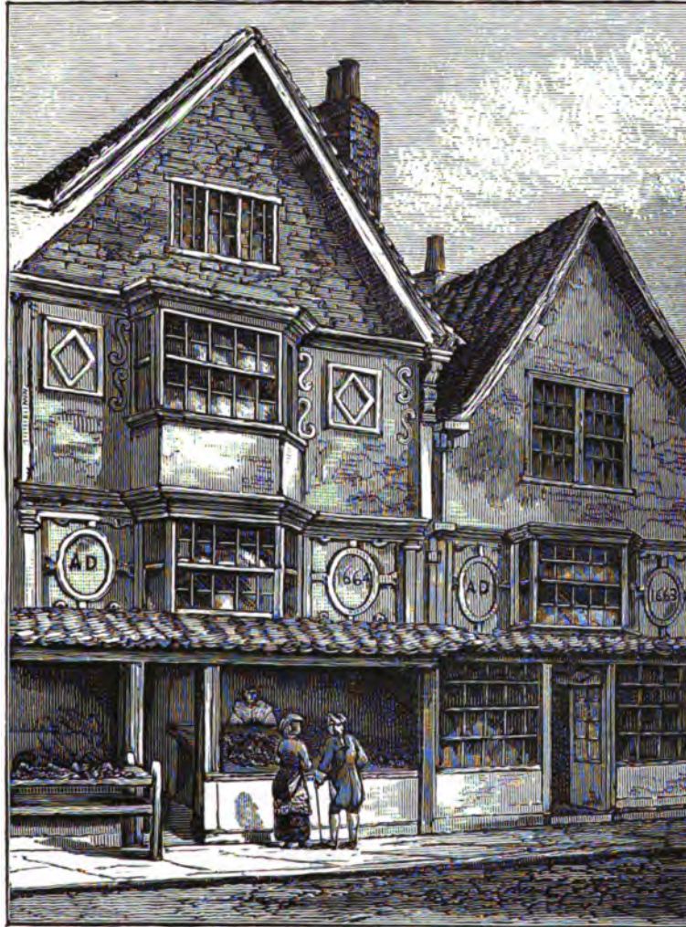
Houses in Peter Street.
